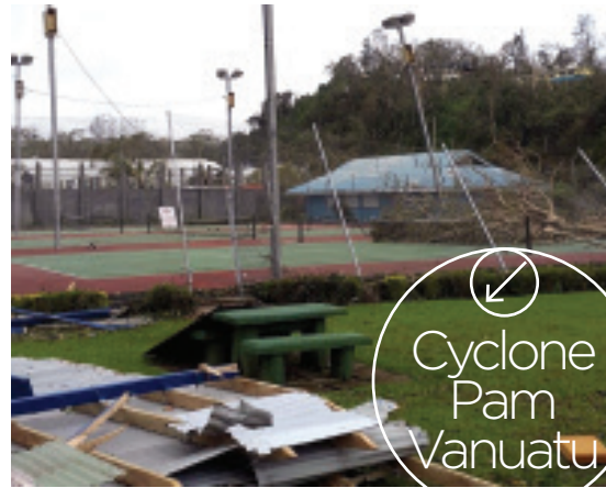
TENNIS CARES ASSISTED IN THE REBUILDING OF THE VANUATU TENNIS CLUB.
