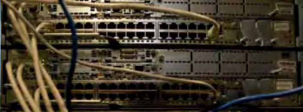
A complete re-build of Tennis Australia's main computer room was undertaken.
