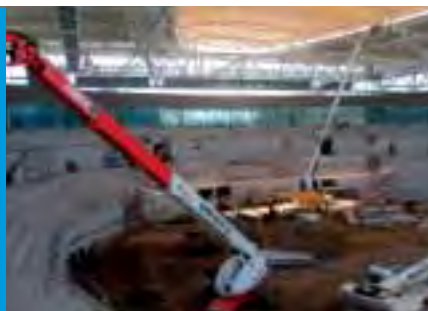
Pre-tournament construction at Pat Rafter Arena.
