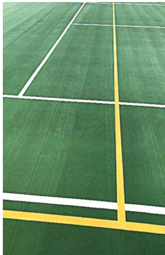
Image 3.1.20 Acrylic court multi-use line marking
