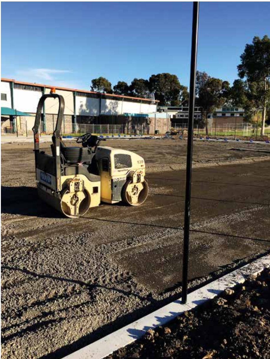
Image 3.1.1 Crushed rock proof roll
