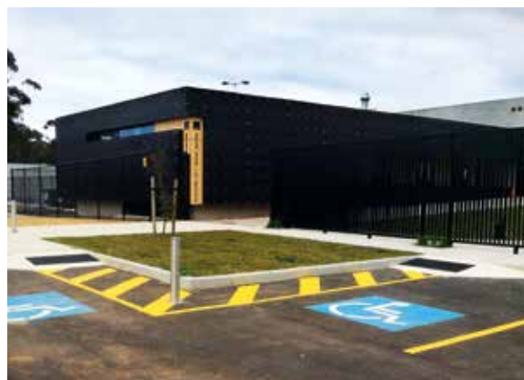
Figure 3.4.4 Accessible clubhouse entrance
