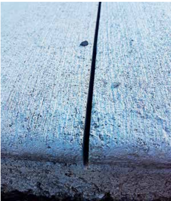
Image 3.1.3 Saw cut joint
